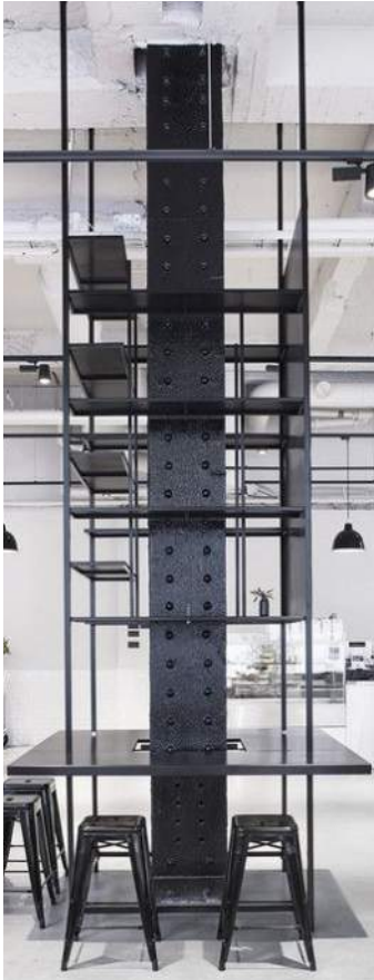
Communal table to wrap around column Custom hot rolled steel shelving to wrap around column and support communal table
